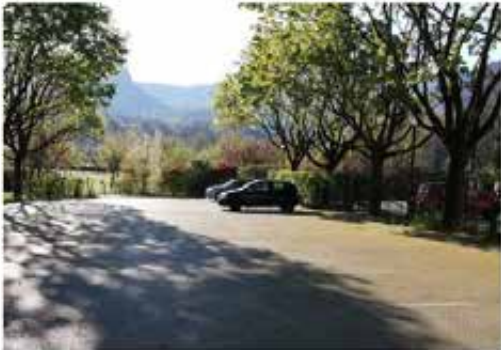
Parking en béton poreux, Beauvoir-en-Royans (illustration)
